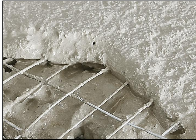
Figure (1.1): Mortar Being Applied to Wire Mesh
